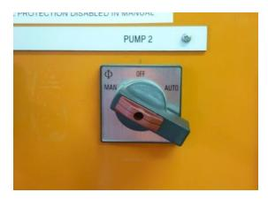
As pump starts running, observe AMP meter reading. Bore Pump 2 AMP meter should read 45 AMPS and green light should indicate Bore Pump 2 is running. Run bore for a minimum of 30 minutes.
