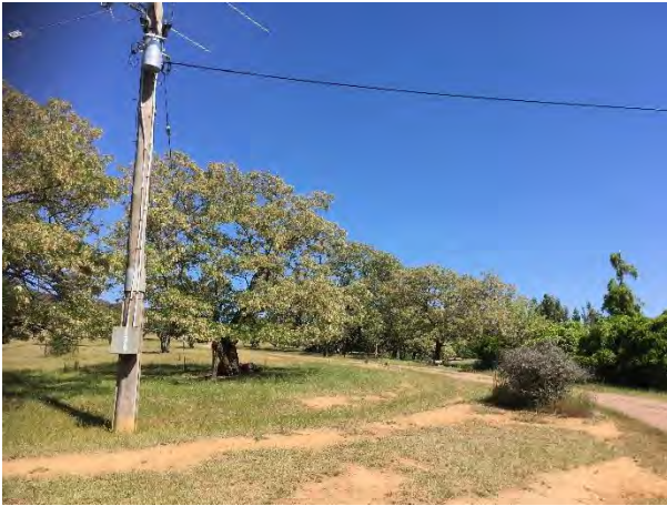
Figure 17 Existing overhead powerline and internal driveway servicing proposed lot 2.
