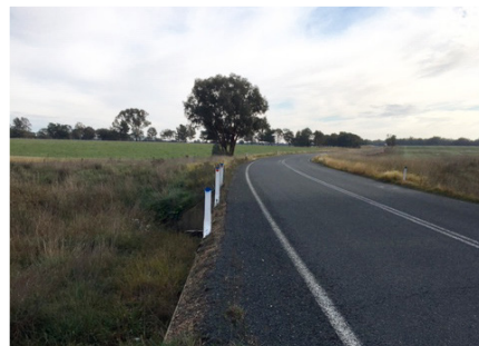
Pic Culvert north of Burrumbuttock.
