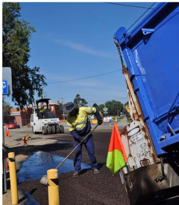
Pic Greater Hume Council Operational Staff working on sealing a road.
