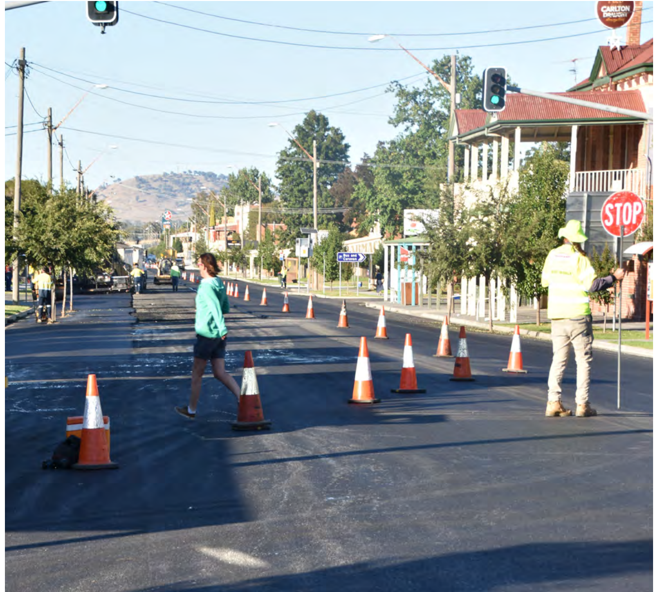
Pictured: Asphalt being installed in Albury Street, Holbrook in March 2018. Roads and Maritime Services funding of $852,916 for pavement upgrade was agreed to by Council to take over maintenance responsibility for the roadway.
