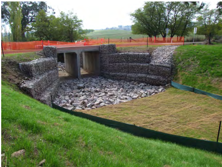
Pictured: Reconstruction of an existing culvert on Sweetwater Road, Mullengandra, tender value $168,514.
