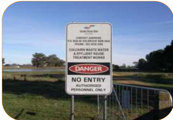
Figure 3: Photos of Signage to Warn the Public of Hazards
