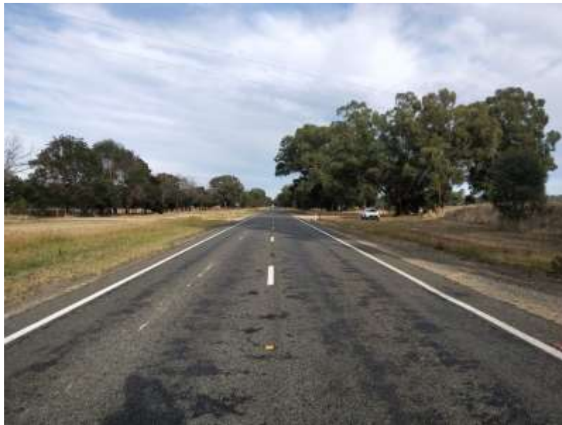
Figure 2-2: Looking west along the Riverina Highway, with Humphreys Road on the right hand side
