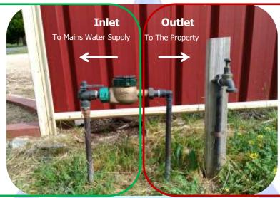
The resident/property owner is responsible for the maintenance and repairs of the pipes from the meter into the house (the outlet side). Contact a plumber if the issue is on this side.
