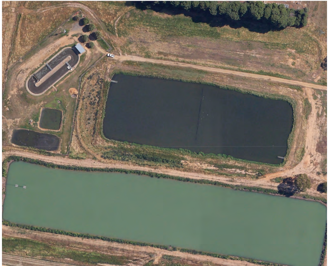
Pictured (above): Culcairn Sewerage Treatment Works
