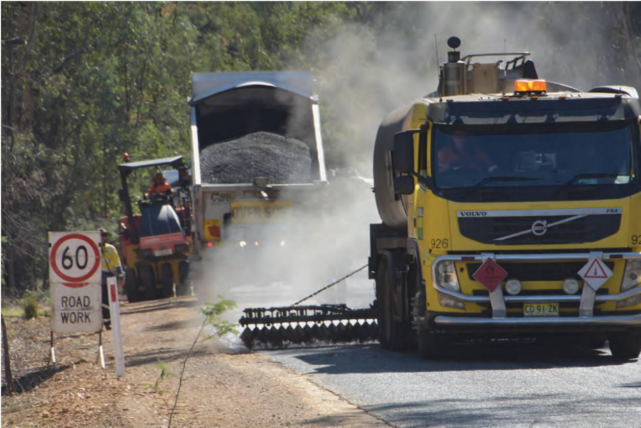
^ Bitumen reseal Mountain Creek Road - April 2020
