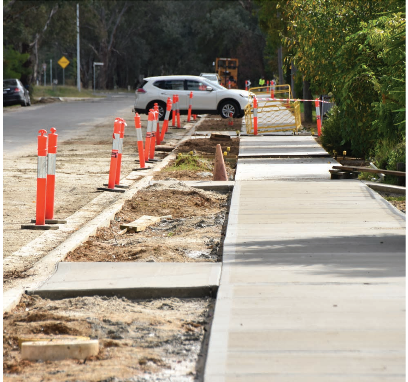
Pictured: New footpath Pioneer Drive, Jindera
