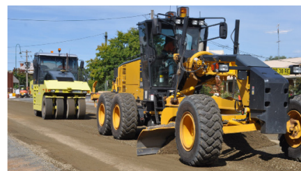
Pic Grader and Roller from Council's fleet of construction equipment
