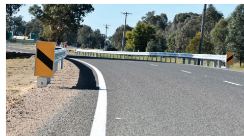
Pic Road reconstruction and widening.
