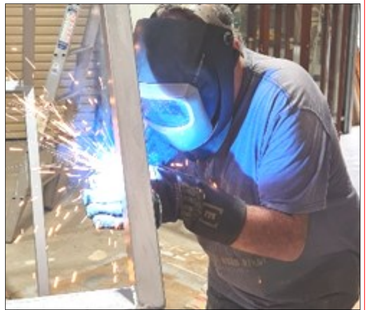
Lance Smith welding frame for “little green shed”.
