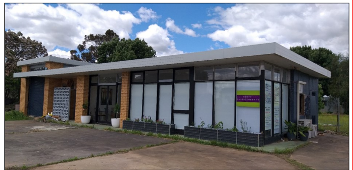
Renovations underway for old servo.
