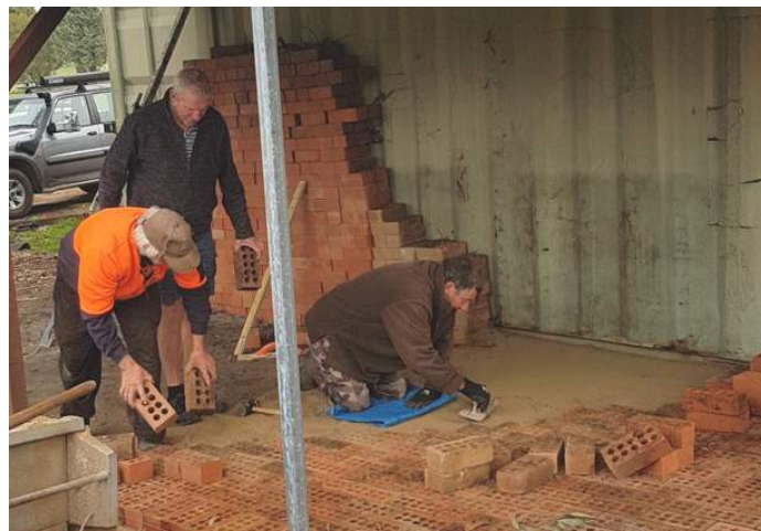
Frank, David & Greg constructing the new golf buggy storage shed
