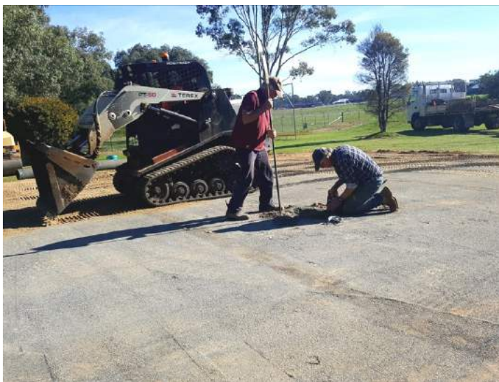
Final work being completed on the greens.
