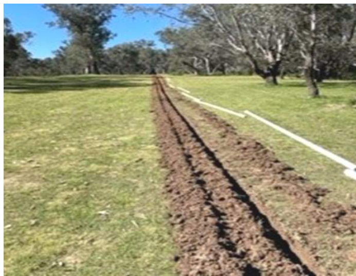
Pat Fuge Back filling Pipes and trenches
