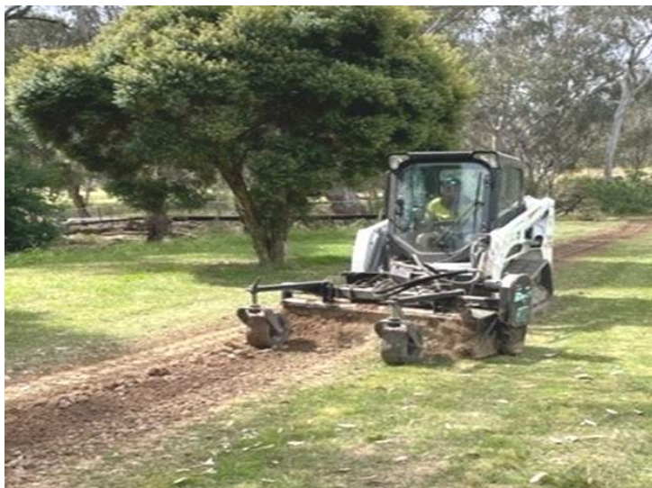
Pat Fuge Back filling Pipes and trenches
