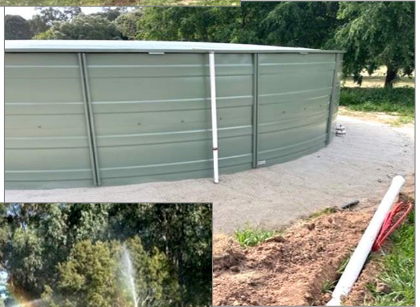
The 220,000 litre tank installed on the 23 rd December 2023
