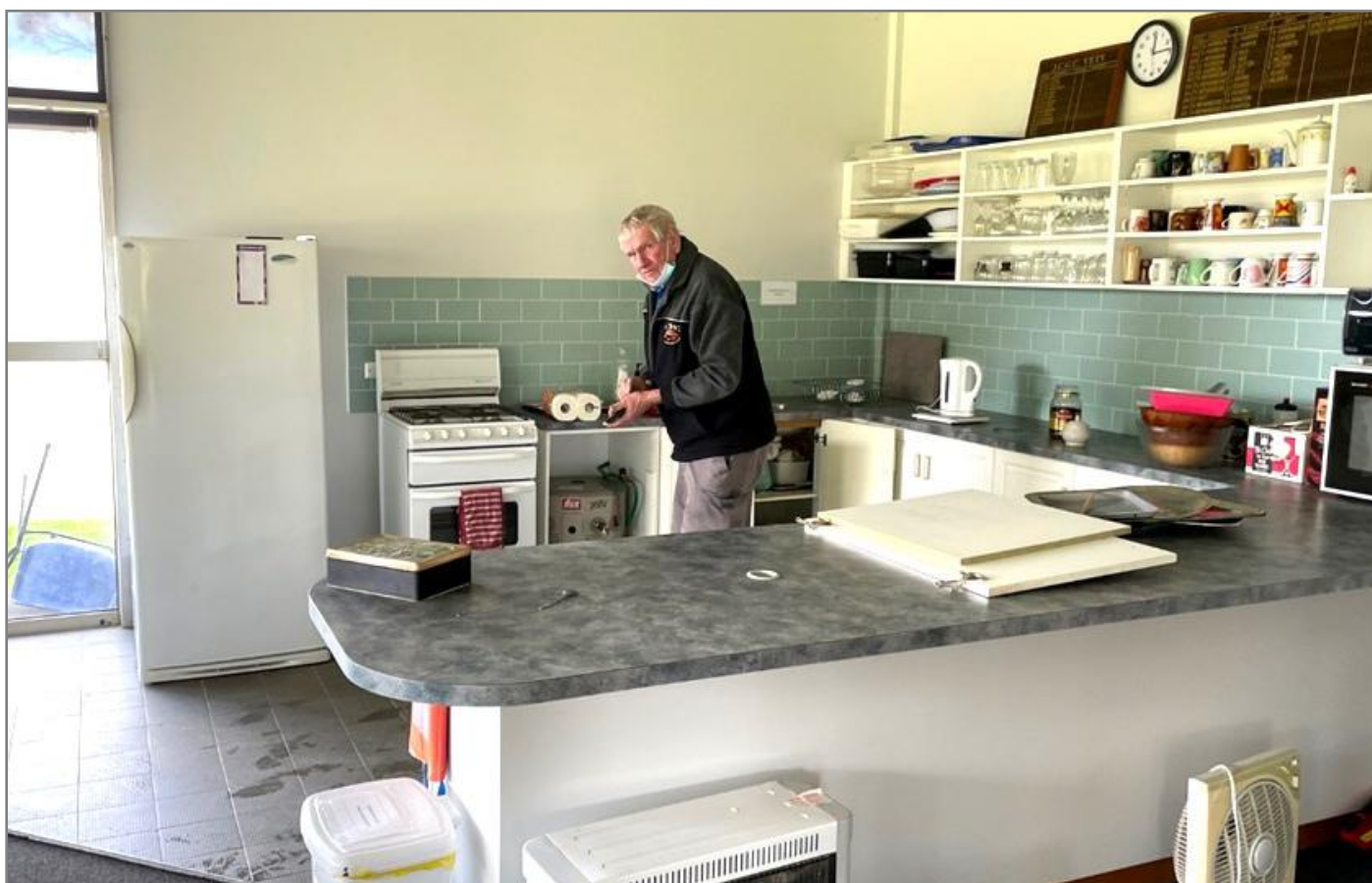
Photo showing Frank Shannon, long time member and one of our – ageing – and committed “grounds committee” at his “second home”, undertaking various repairs to the clubhouse including fixing leaking hot water service, blocking mouse entry holes and numerous other tasks that nobody thinks about.
