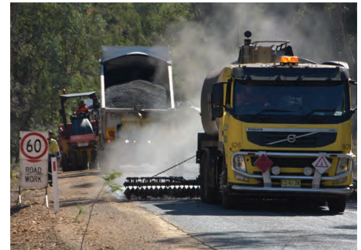
^ Bitumen resaling Mountain Creek Road, April 2020
