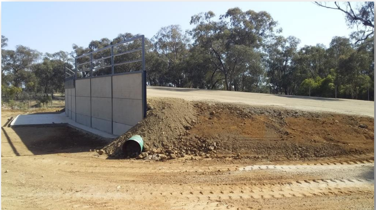
Pic: Brocklesby Transfer Station 1
