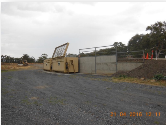
Pic: Henty Transfer Station 1
