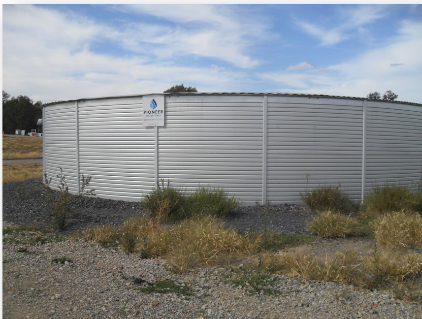
Pic: Waste Water Storage Tank Holbrook
