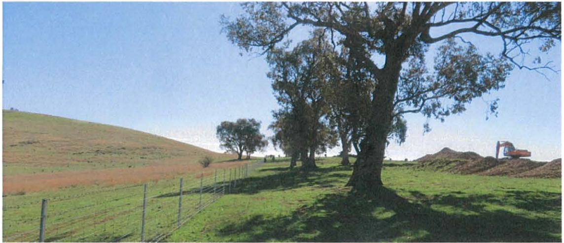
Photo 1. Looking westerly along adjoining Lot 2 DP117528 being former road reserve. The extraction site is located to the right.
