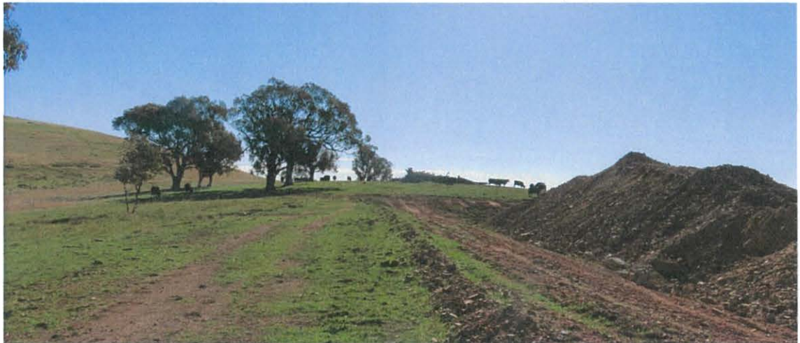
Photo 2. Looking westerly along western edge of development site.
