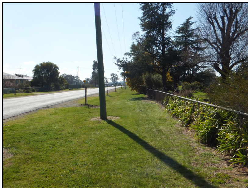
Photo 3 existing typical section of Lookout Road NE verge for construction of WSP in Option 1 also refer Photo 4 below
