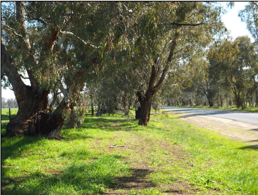
Photo 1 existing typical timber section of Lookout Road on NW verge for construction of WSP
