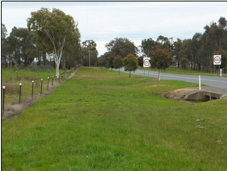
Photo 7 shows existing section of Lookout Rd on NW verge at floodway for construction of WSP as described in Section 3.2
