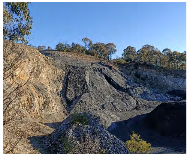
Figure 14 View of existing quarry pit and work area.
