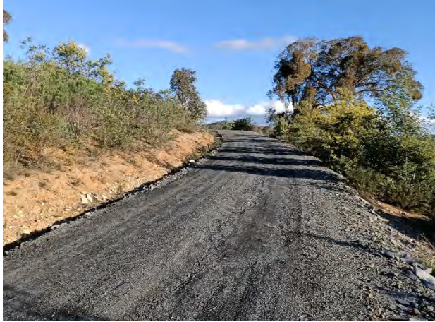
Figure 3 Entrance to site from the Holbrook-Jingellic Road.
