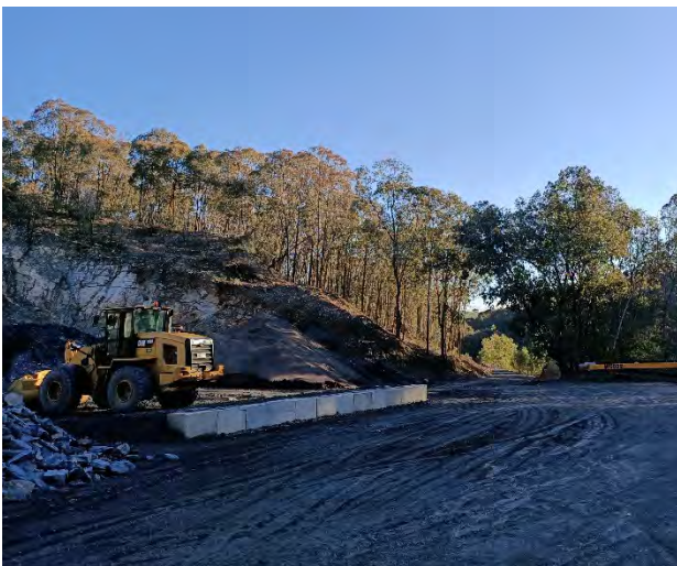
Figure 13 View of existing quarry pit and work area.
