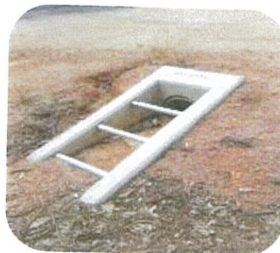
Typical Winged Headwall and Pipe Used on Rural Roads
