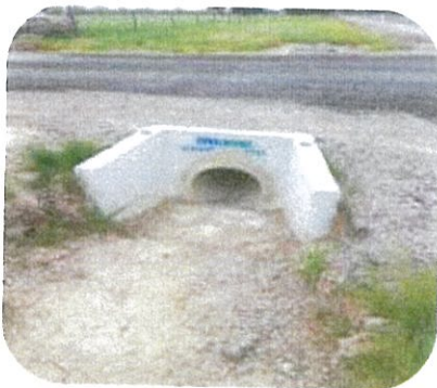
Typical Winged Headwall and Pipe Used on Rural Roads
