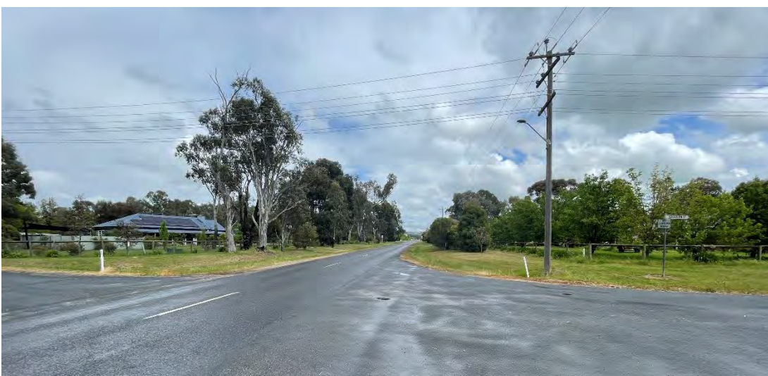
Figure 10 – View looking west on Adams Street towards the intersection with Goulburn Street
