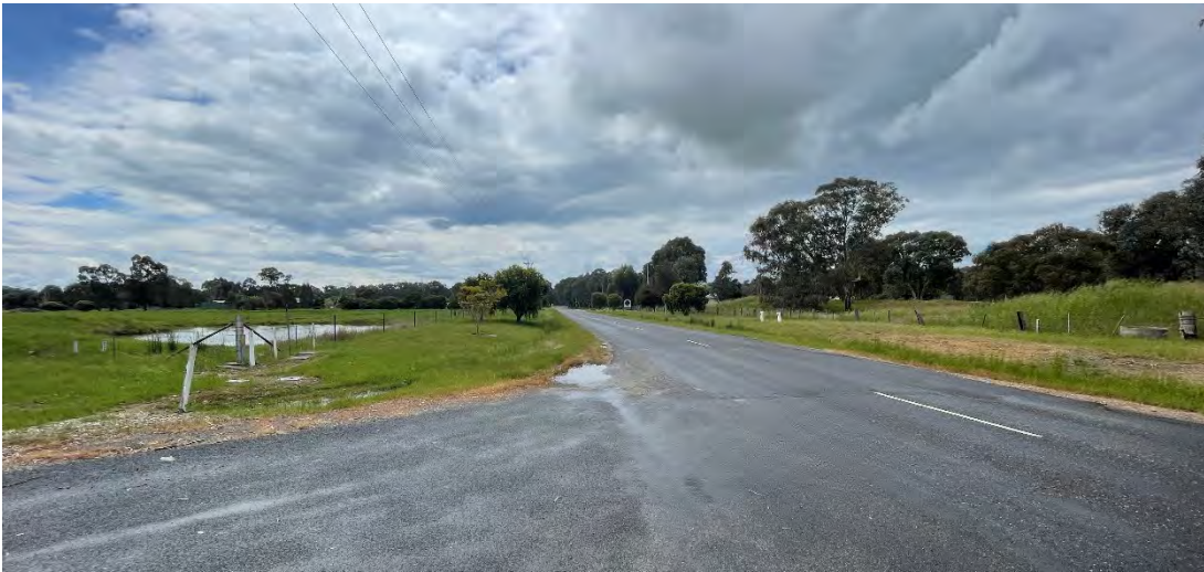
Figure 11 – View looking east on Adams Street towards the intersection with Goulburn Street
