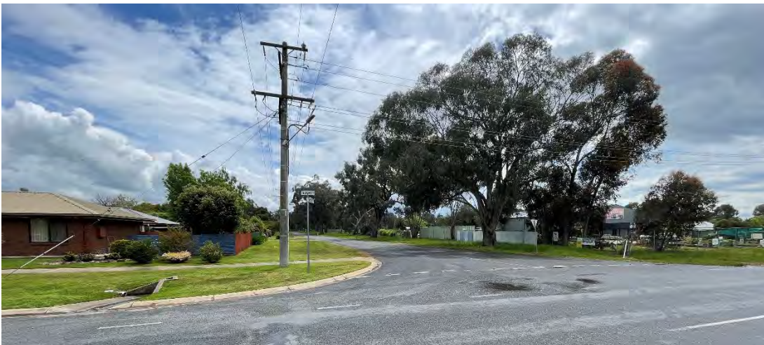
Figure 15 – View looking north on Adams Street towards the intersection with Mitchell Street
