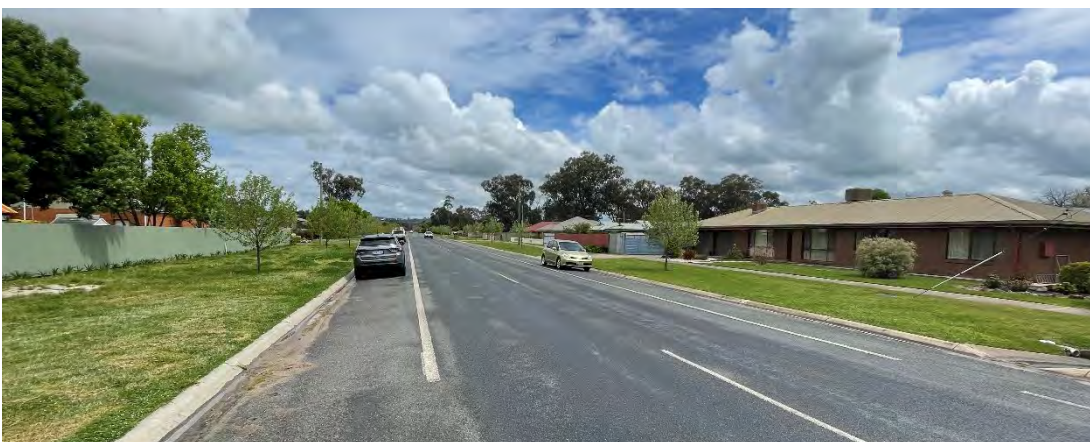
Figure 16 – View looking west on Adams Street from the intersection with Mitchell Street
