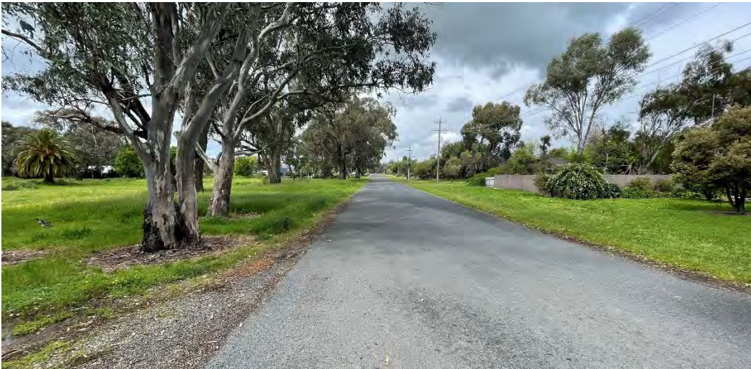
Figure 14 – View looking south on Mitchell Street from the front of the southern parcel
