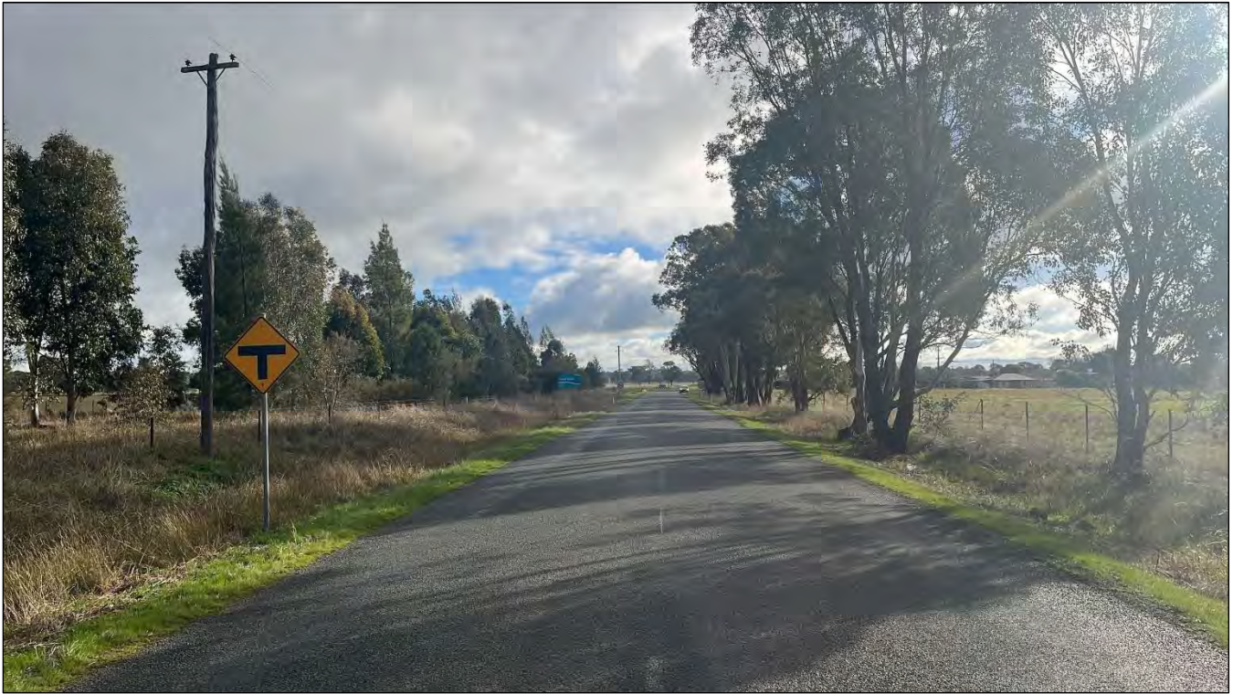
Figure 5: Walla Walla Road facing west towards the T-intersection with Commercial Street
