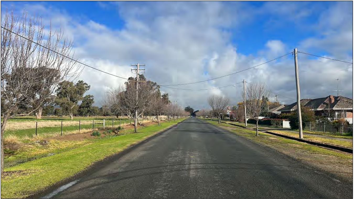
Figure 3: Commercial Street facing south
