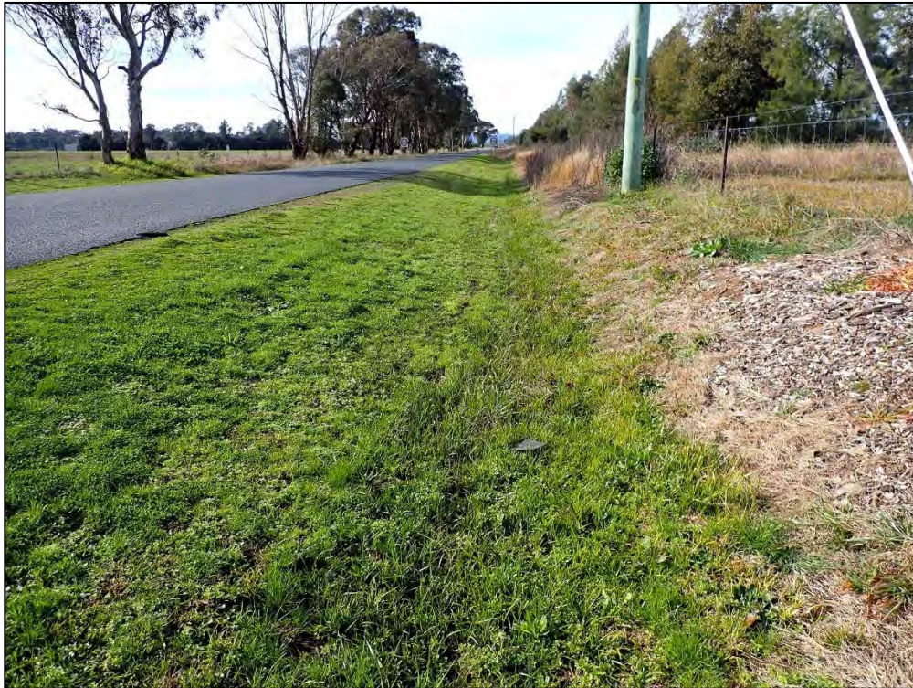
Plate 1: View east of drainage channel along southern-most side of Walla Walla Road transport corridor.
