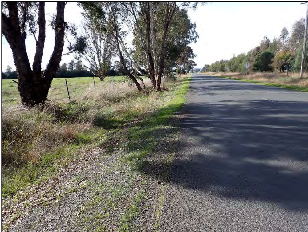
Plate 2: View east of drainage channel along northern-most side of Walla Walla Road transport corridor.
