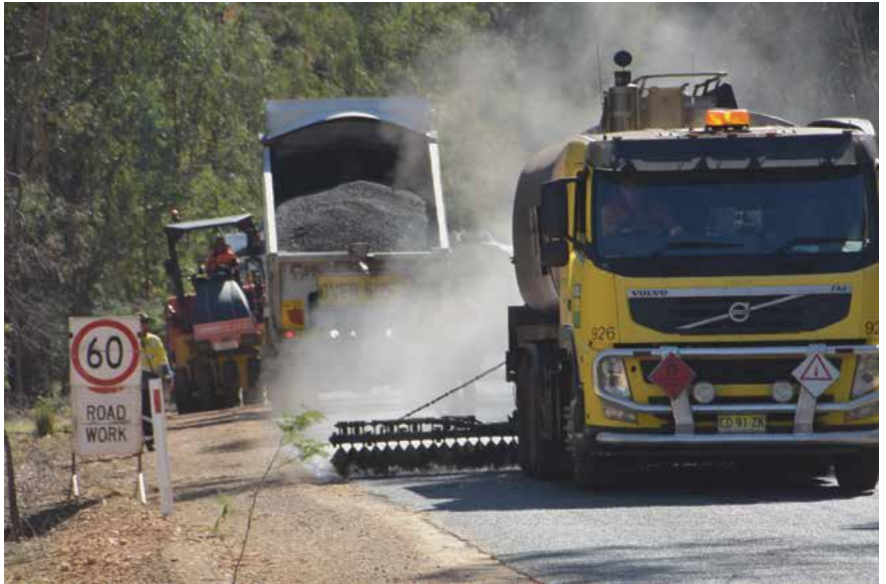
^ Bitumen reseal Mountain Creek Road - April 2020
