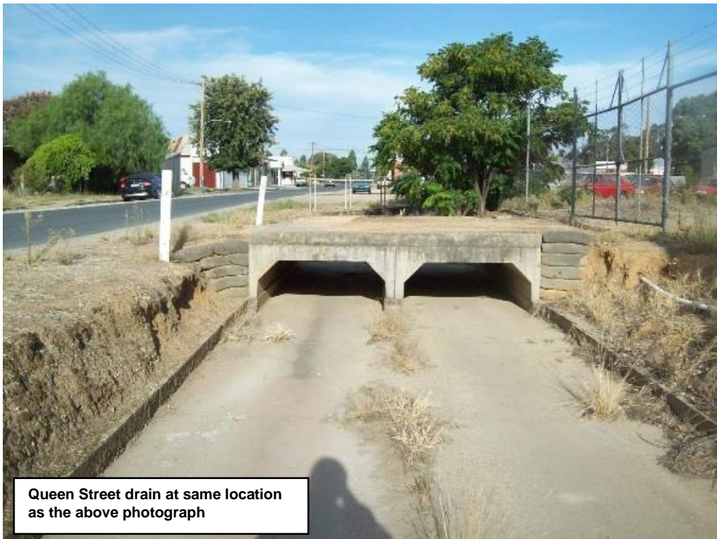
Figure 4 Queen Street Drain
