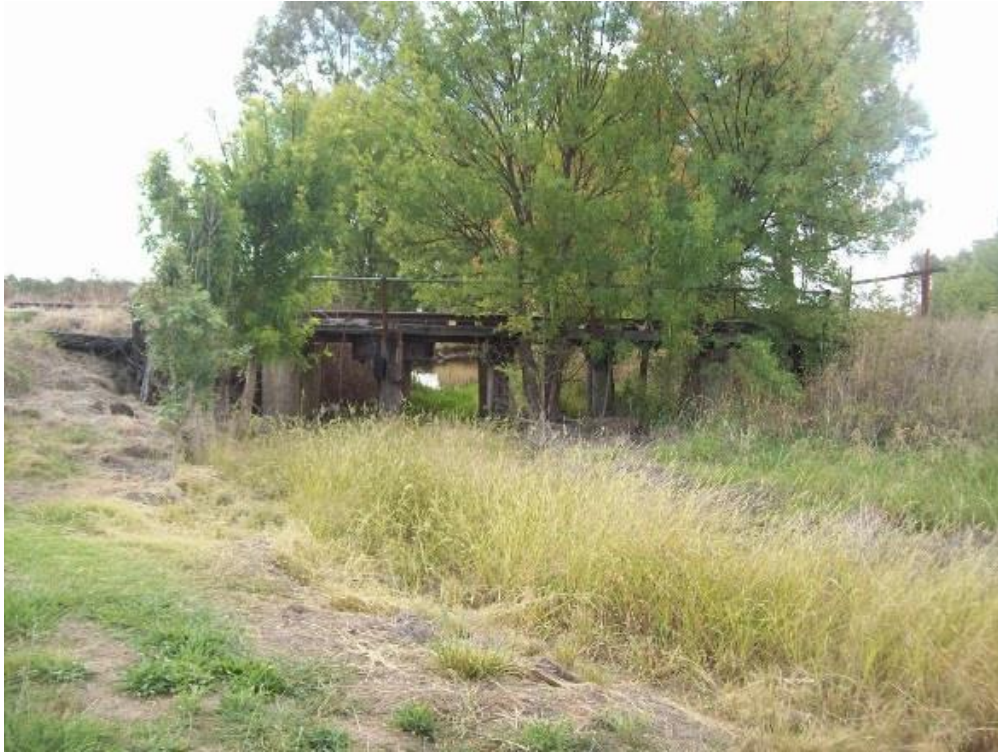
Figure 10 Railway Bridge at Walla West Waterway
