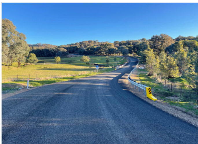
Pic Ferndale Road, Woomargama. Widening, sealing and improved transverse drainage completed.
