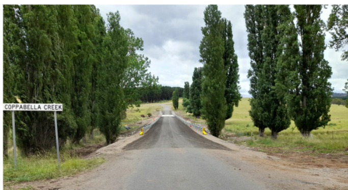
Pic Reconstructed Coppabella Bridge, Coppabella.
