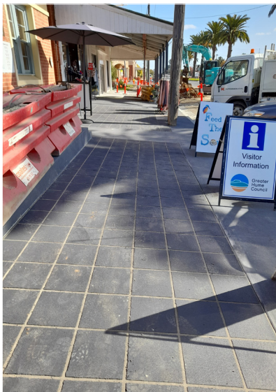
Pic New paths, kerbing and guttering are part of the Culcairn Business District upgrade.
