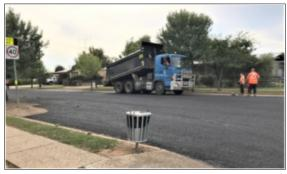
then the truck with blue metal went backwards where the tar was, then workers with brooms swept the new surface where necessary, to make a smooth surface. Normal traffic was disrupted for only a short time. It was a highly organised activity. Hopefully very little tar went onto cars as they were driven on the new surface.
