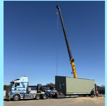
Big crane at MBI engineering lifting a switch-room to be taken to site in Ballarat.
